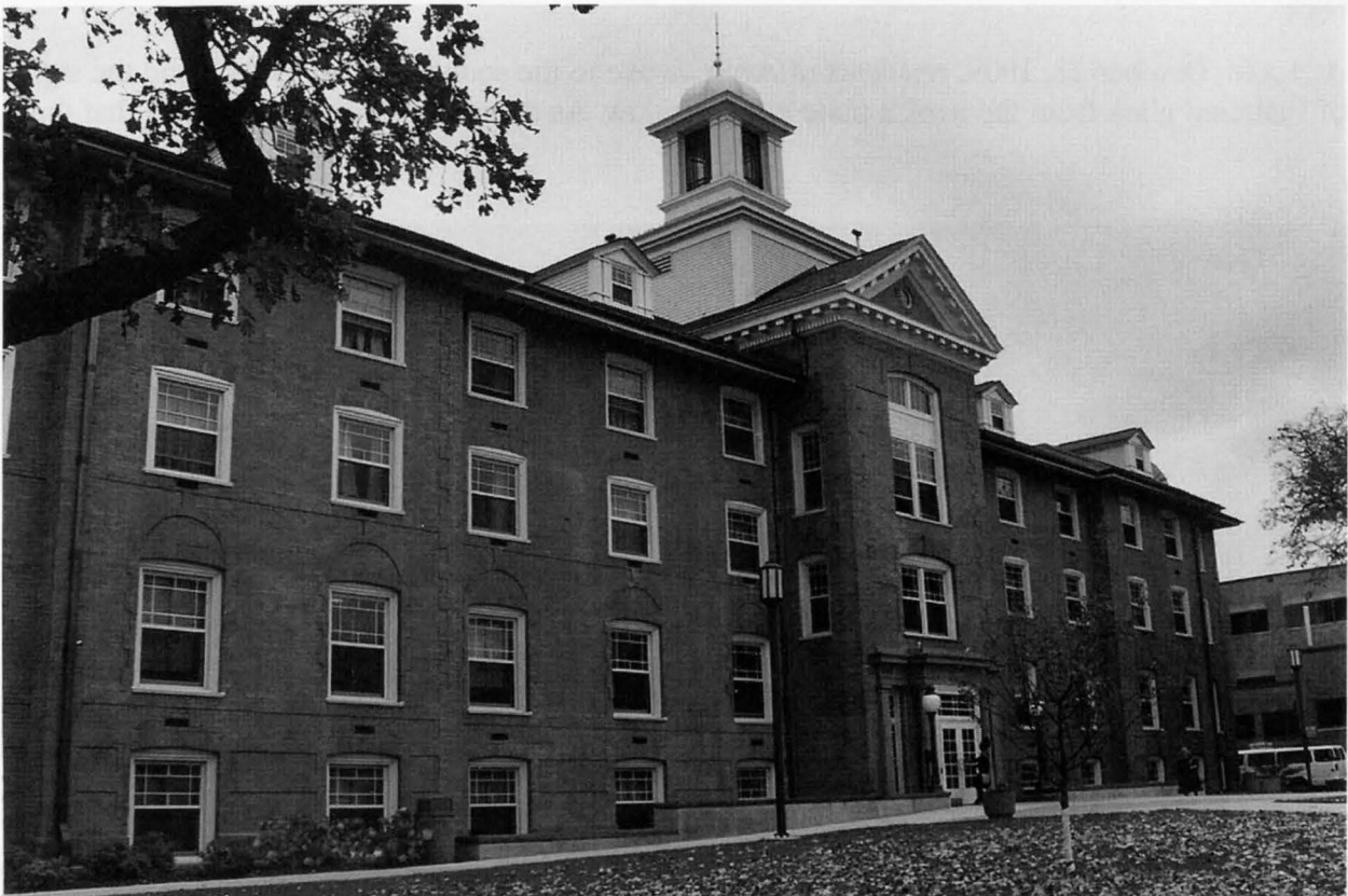
Lawrence Hall is one of four vintage buildings on the St. Cloud State University campus. The structure was rebuilt in one year after a disastrous 1905 fire.
