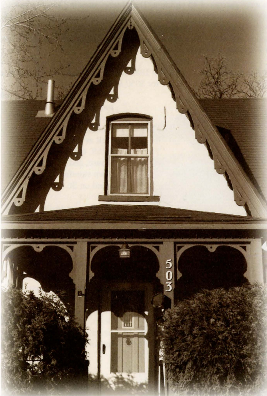
Bargeboards grace the central gable of the Gingerbread House. A bargeboard is an ornately-carved board nailed to the projecting edge of a gable or porch.
