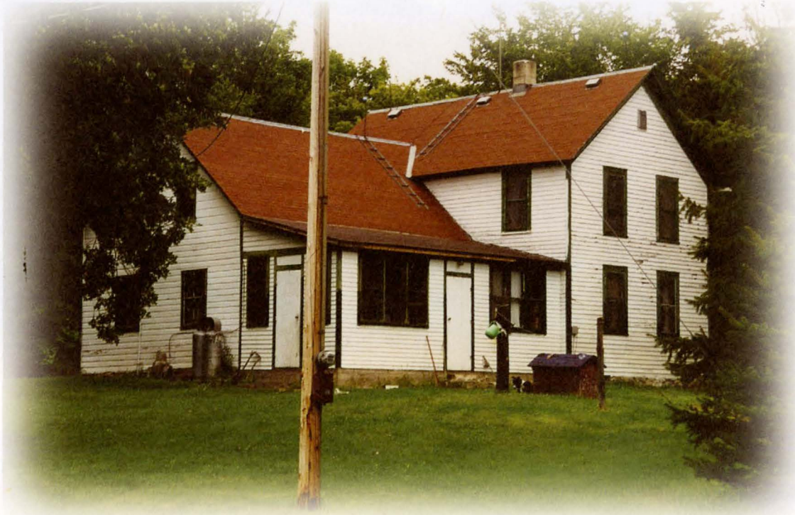
The Gogala farmhouse near St. Anthony is an L-shaped Greek Revival home. The first portion was built in the early 1880s by Anton Gogala, Sr. A framed bay was added in 1916. Today, both sections are clapboard-sided and painted white with cornerboards trimmed in green.
