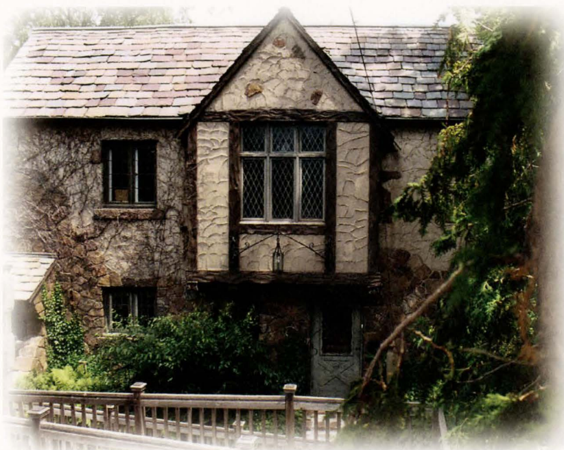
The façade of the Brower House shows leaded glass windows, hand-tooled beams, and a decorative exterior stucco finish.
