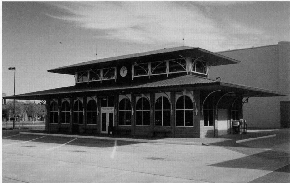
The Metropolitan Transit Center in downtown St. Cloud is done in a style resembling the Victorian metal-and-glass train sheds found in England and in Europe.
