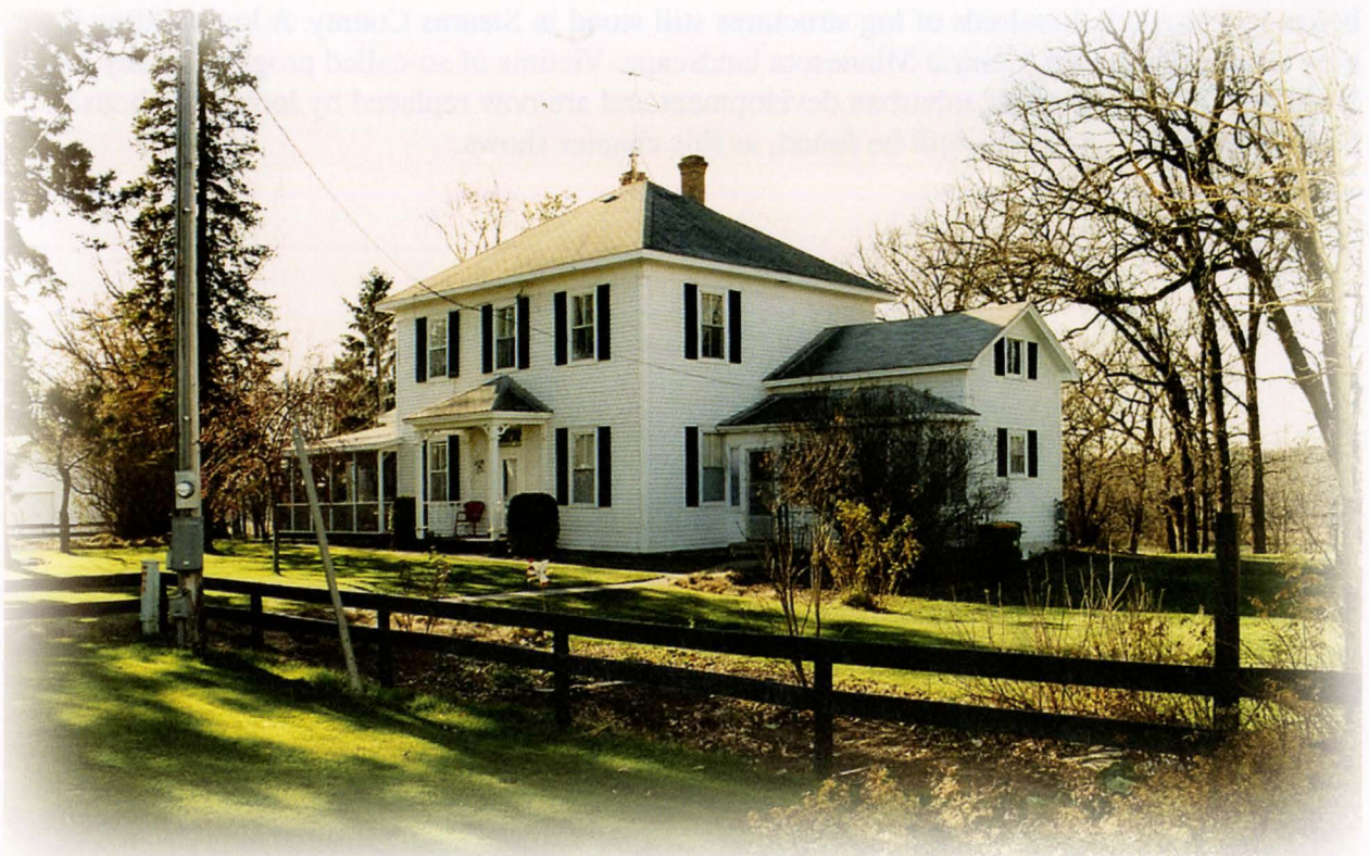
Built in 1856, the Georgian Revival Lorenz farmhouse faces Yankee Road in Rockville Township.
