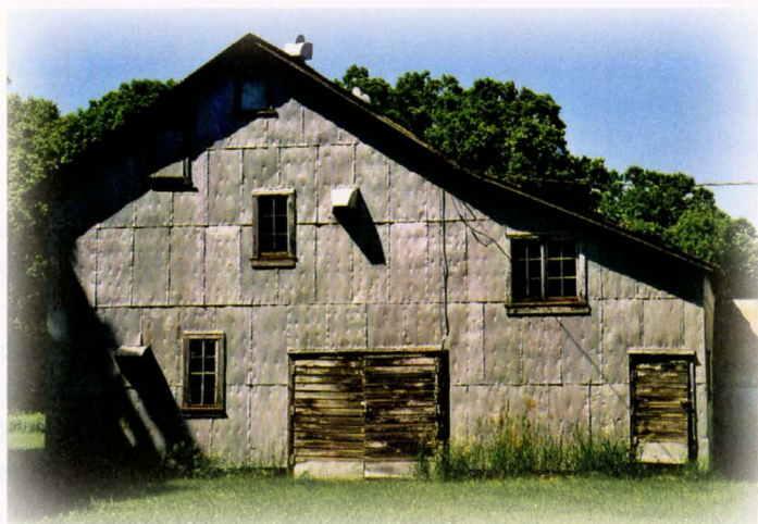
The metal siding on the Graves' barn is a fine example of salvage architecture.
