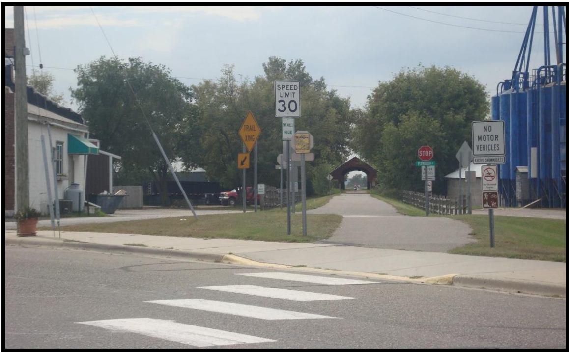
Figure 10. Covered bridge over the Wobegon Trail and Two Rivers River.
