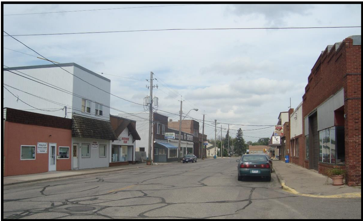
Figure 8. North facing view of main street's streetscape.
