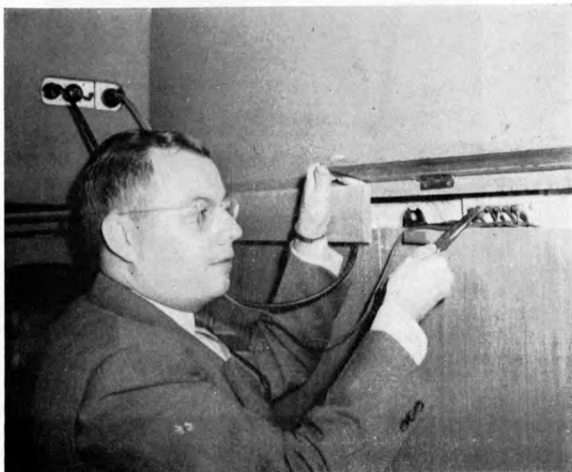
Position of Wiring in Molding
