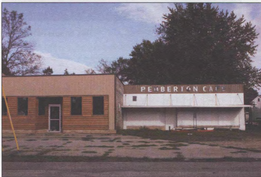
Remains of the Pemberton Café and gas station on Main Street
