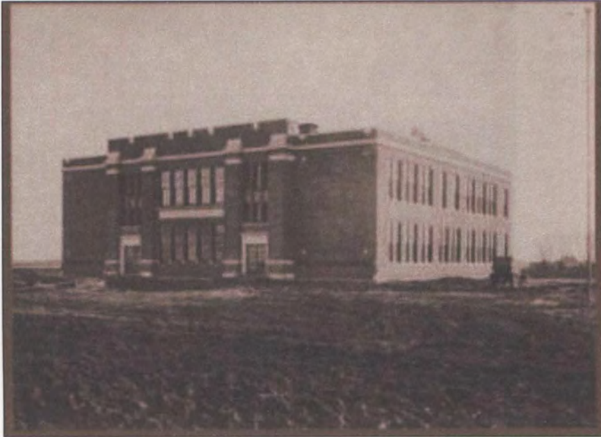
Pemberton School Building around 1920
