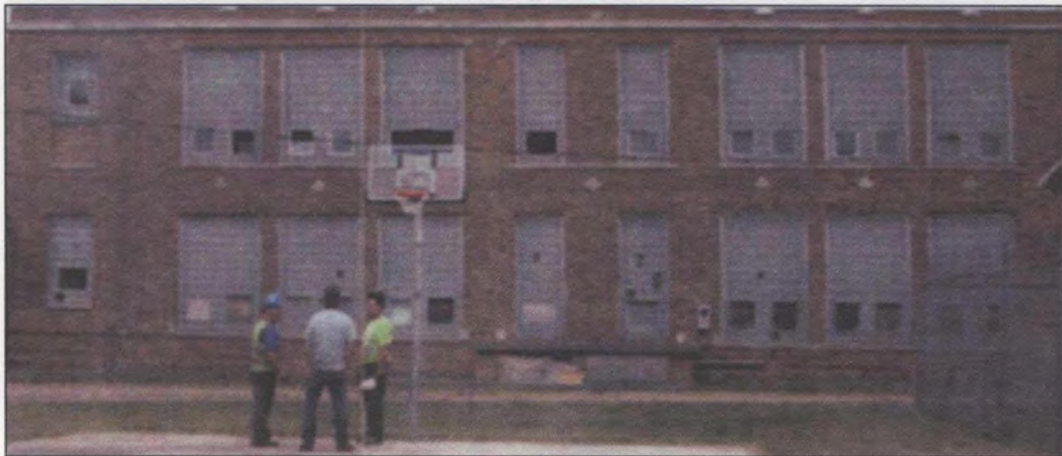
1920 section of the Pemberton School building prior to demolition
